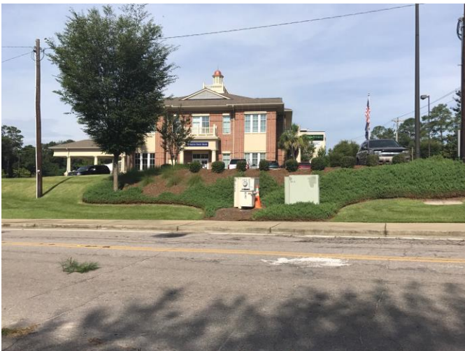
South State Bank – Across from 1514 Brentwood
